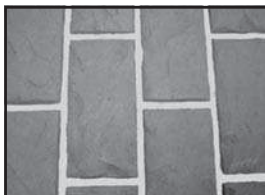
Running Bond Ashlar Stone
